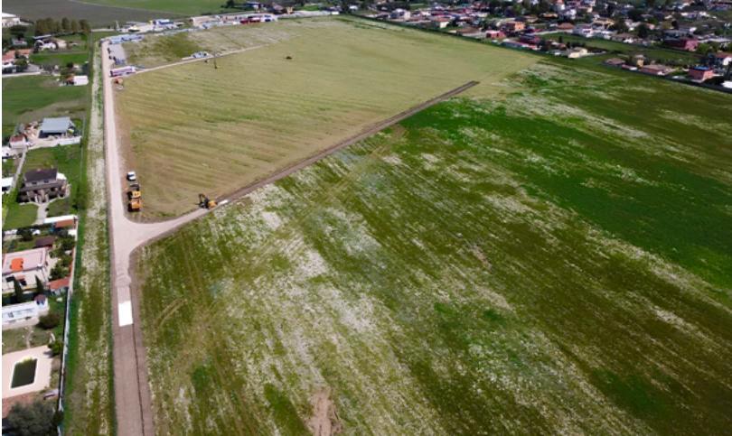
Aerial view of the site of the Latina solar power farm.
