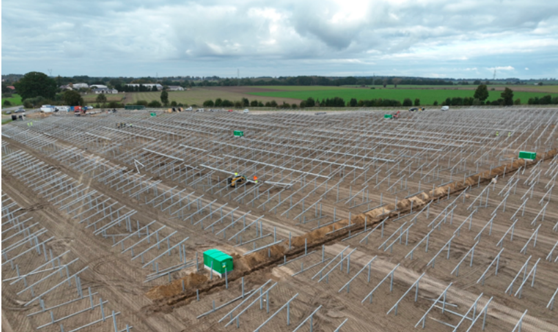
Installation of the solar panels under way at the Resko site.
